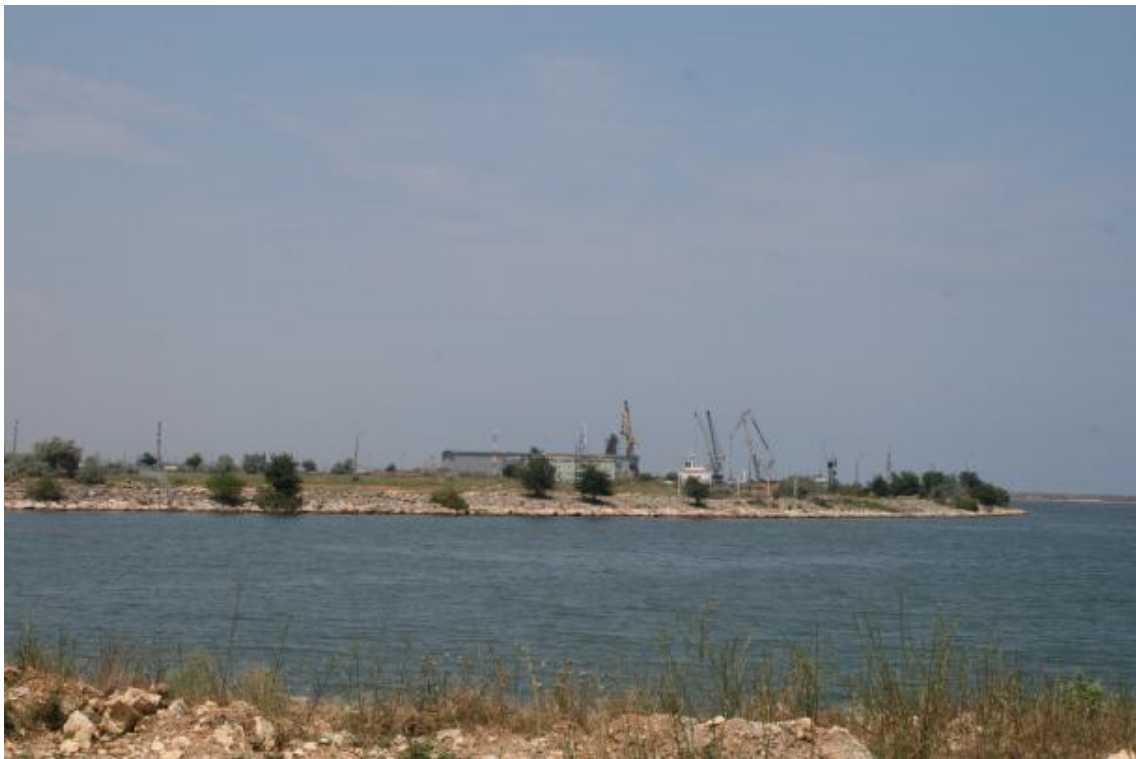
Figure 33 – View from Plot 2 towards AGN3 site
